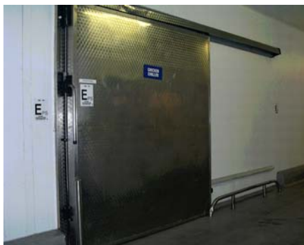
Sliding door labels, note the position of the right hand label at the limit of the 'slide'
