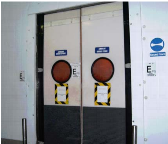
Typical labelling, the panels the other side of the door have expanded polystyrene cores
